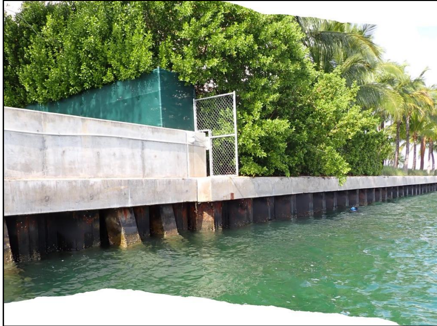
Photo 22: Section 8 stem wall termination and construction change at STA 3+09, looking southwest
