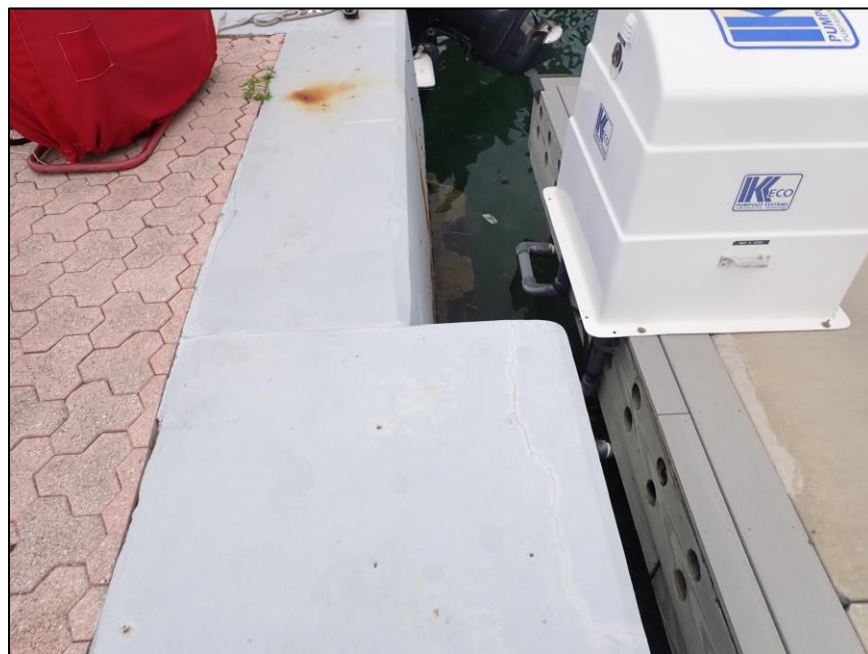
Photo 7: Section 3 reduction in cap width at offshore face, at approximate STA 3+20
