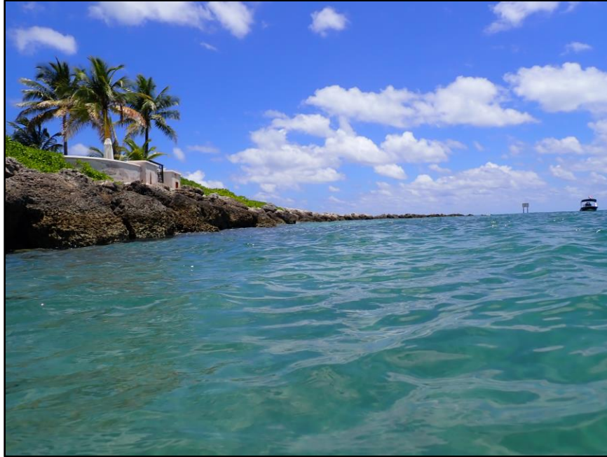
Photo 1: General view of Section 1 breakwater, looking southeast
