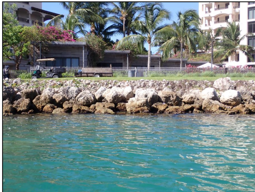
Photo 42: Section 13 Smaller diameter limestone STA 0+00 to STA 8+90
