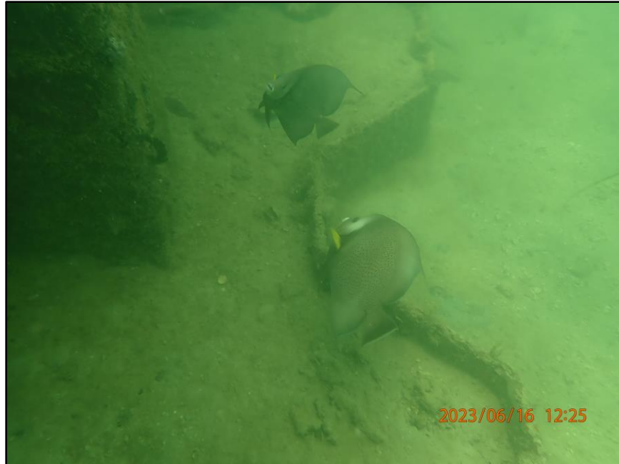
Photo 18: Steel sheet pile toe wall along the base of the Section 6 bulkhead
