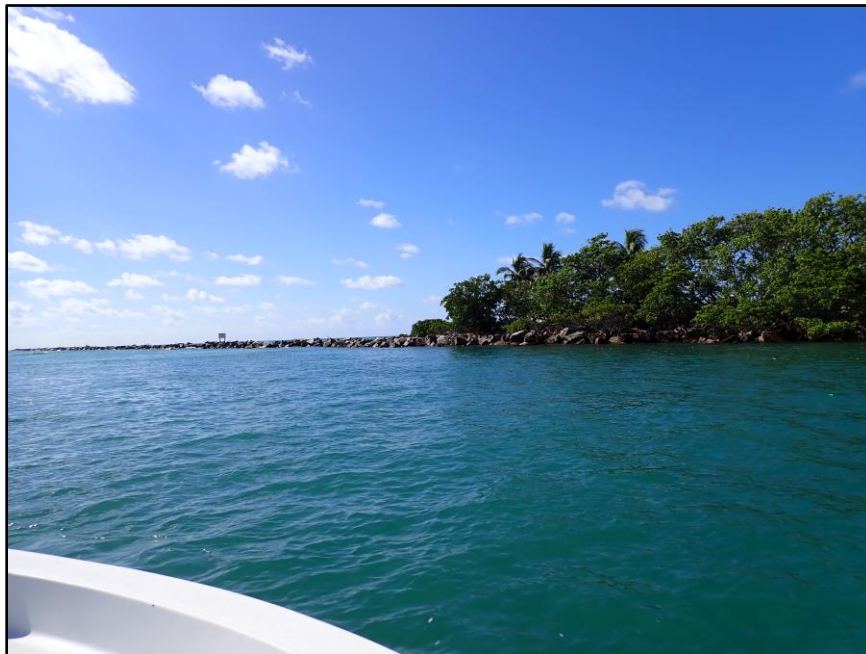
Photo 44: General view of breakwater beyond eastern limit of Section 13
