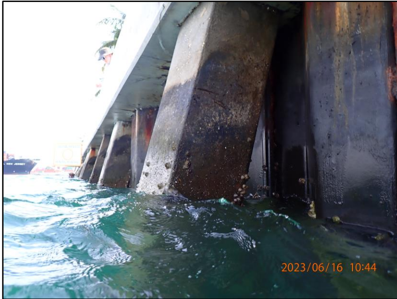
Photo 24: Typical view of Section 8 bulkhead, STA 6+64 to STA 11+69, facing north
