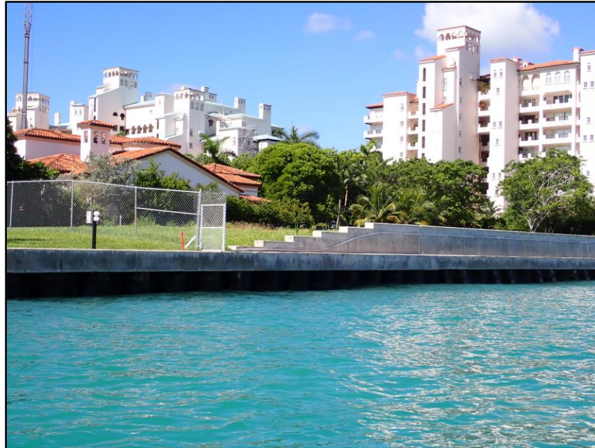
Photo 21: Stepped stem wall at interface between Sections 8 and 9
