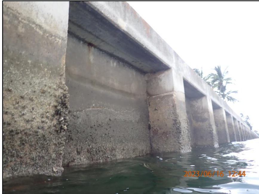
Photo 16: Typical view of Section 6 bulkhead construction
