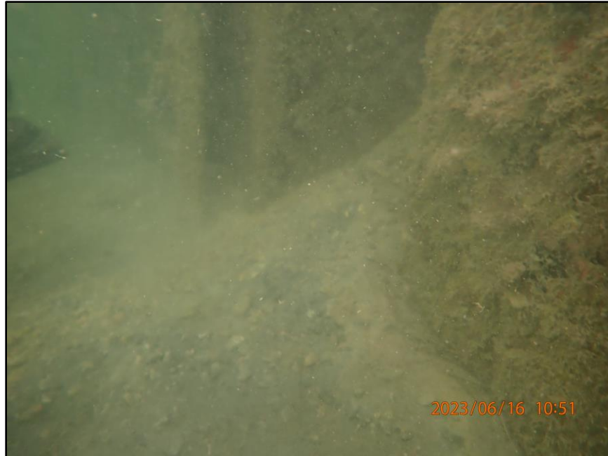
Photo 72: Sediment accumulation at Section 8 termination
