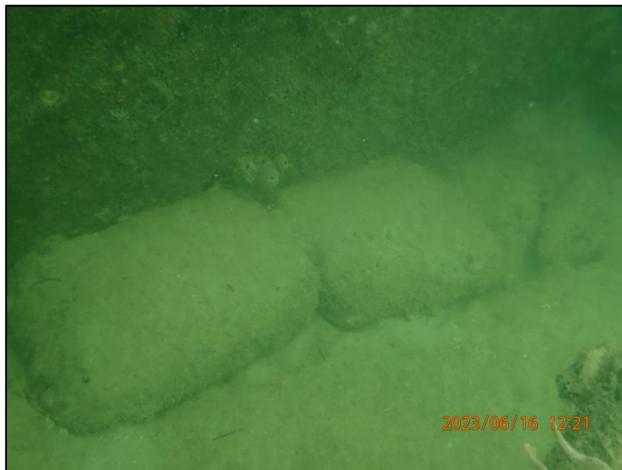
Photo 17: Intermittent grout bag installation along the toe of Section 6
