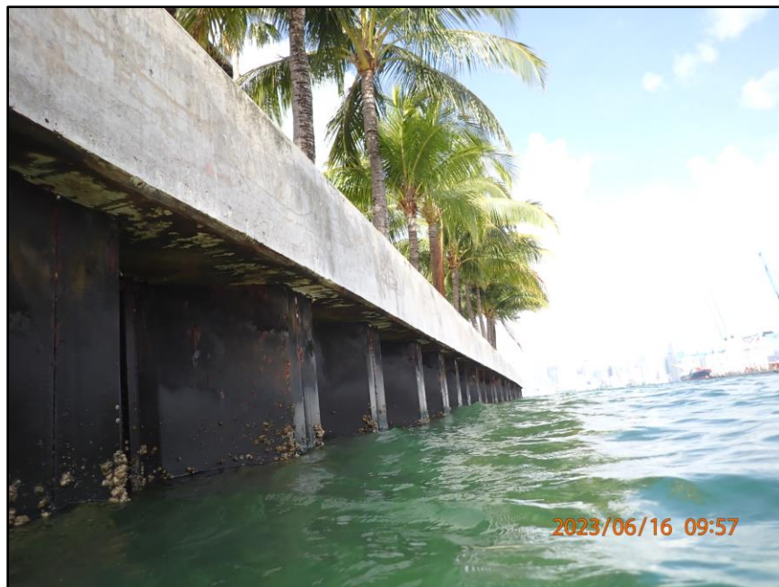
Photo 23: Typical view of Section 8 bulkhead, STA 3+09 to STA 6+64, facing west
