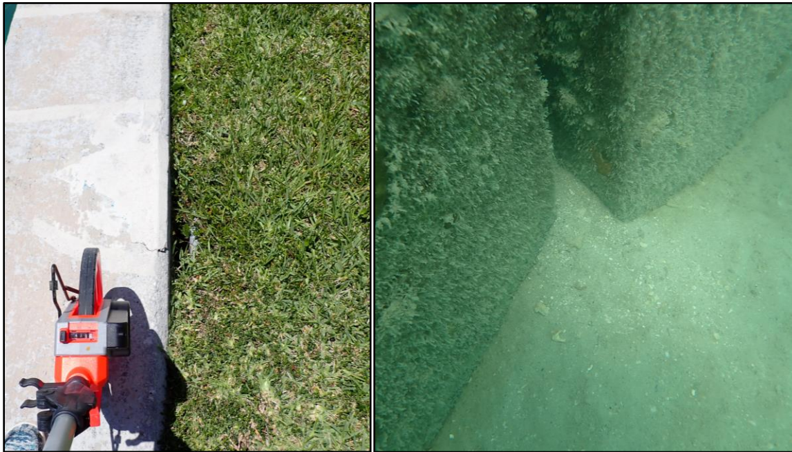
Photo 58: Section 4 Typical view of upland sinkhole in line with sediment accumulation at mudline
