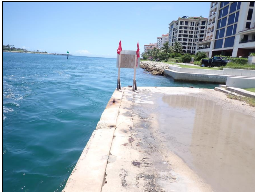
Photo 41: Topside view of Parcel 15
