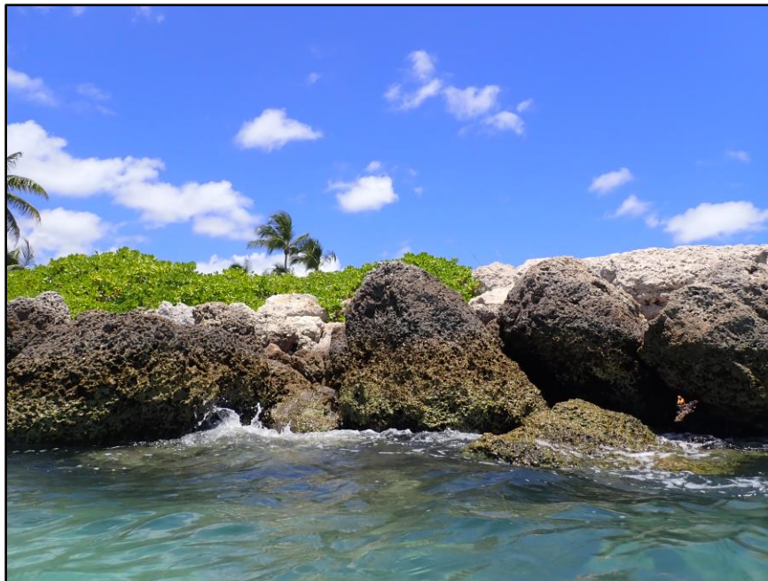
Photo 2: Typical 2-6 ft diameter rip rap along Section 1
