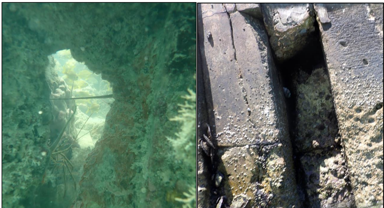
Photo 62: 1 ft deep sinkhole at Section 5 STA. 0+00 E (left) with exposed tie rod attached to Section 4 bulkhead (right)
