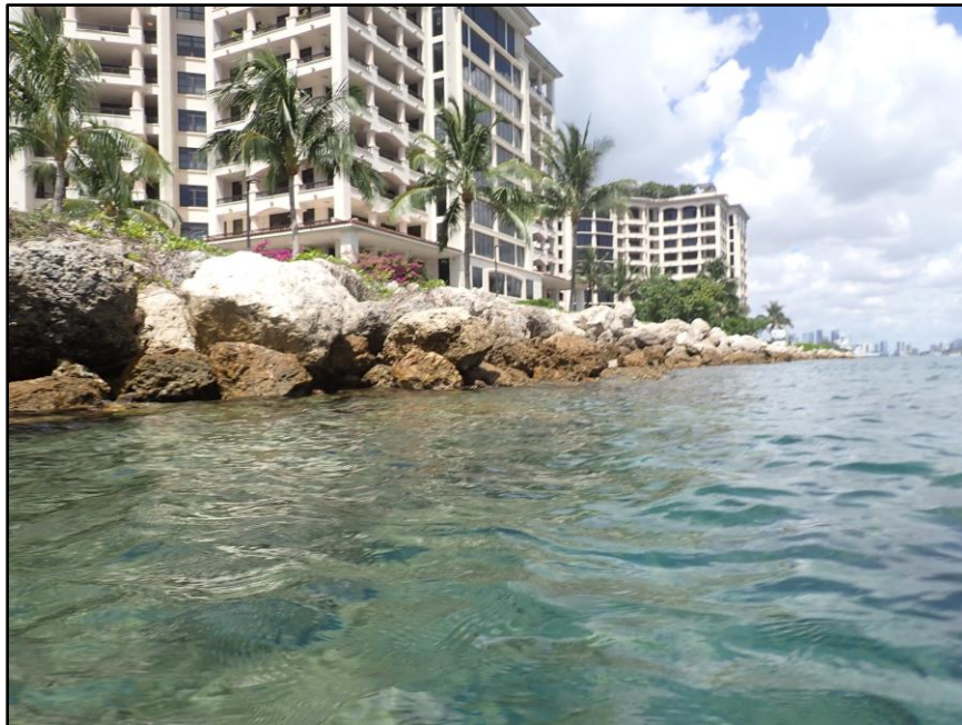
Photo 102: Intermittent grades of smaller diameter riprap at steeper than 1:1 slope
