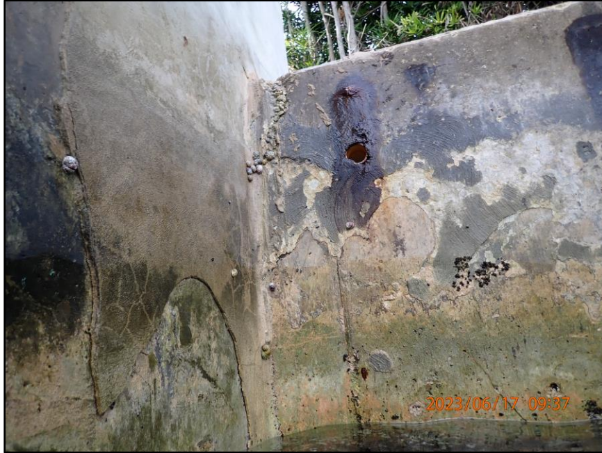
Photo 31: Section 11 change in concrete cap construction at STA 0+84 interface
