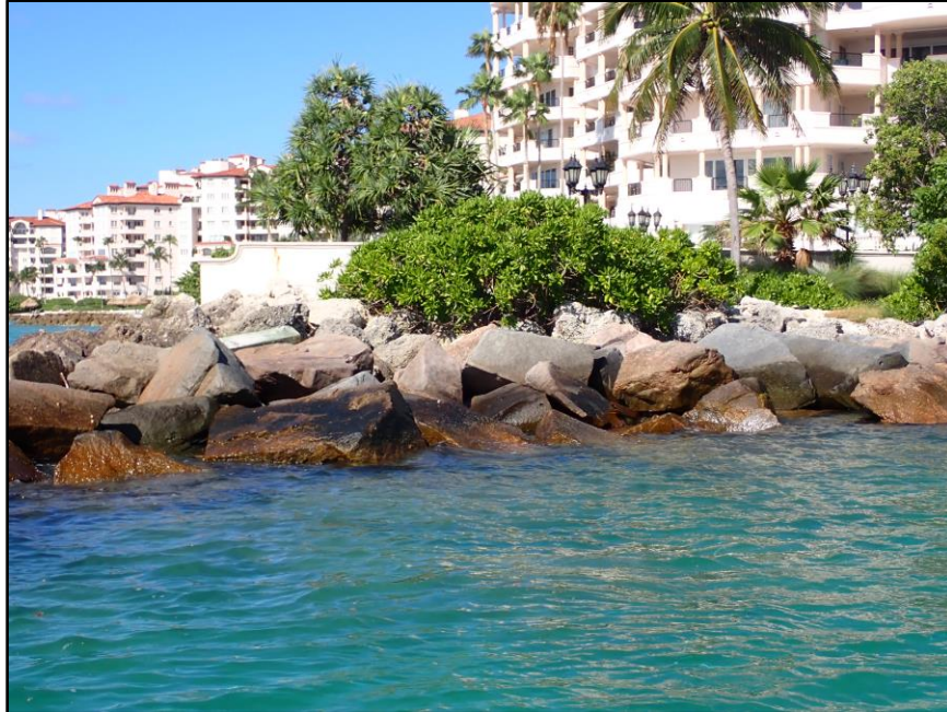
Photo 43: Section 13 Large angular granite stones STA 8+90 to end of breakwater
