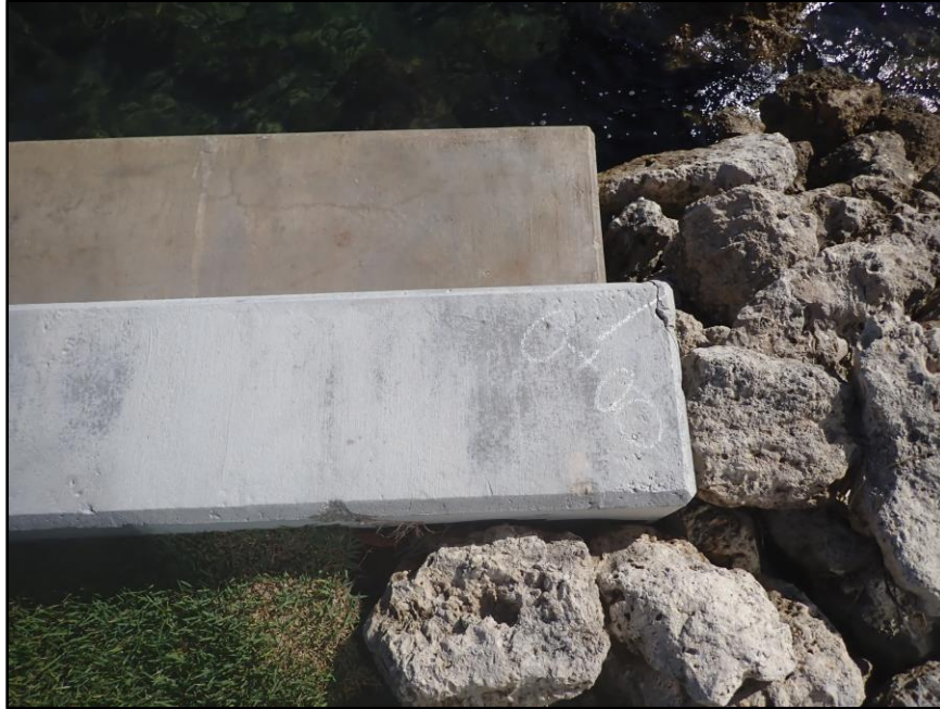
Photo 38: Northeastern termination of Section 12 bulkhead into Task 2 riprap revetment
