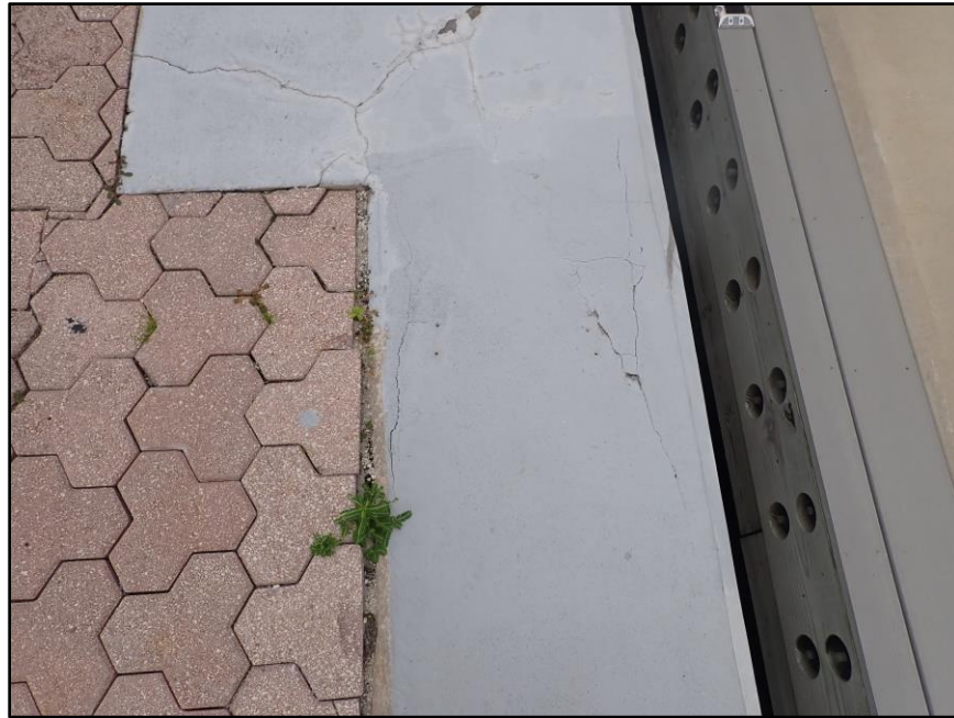
Photo 6: Section 3 increase in cap width at approximate STA 2+60
