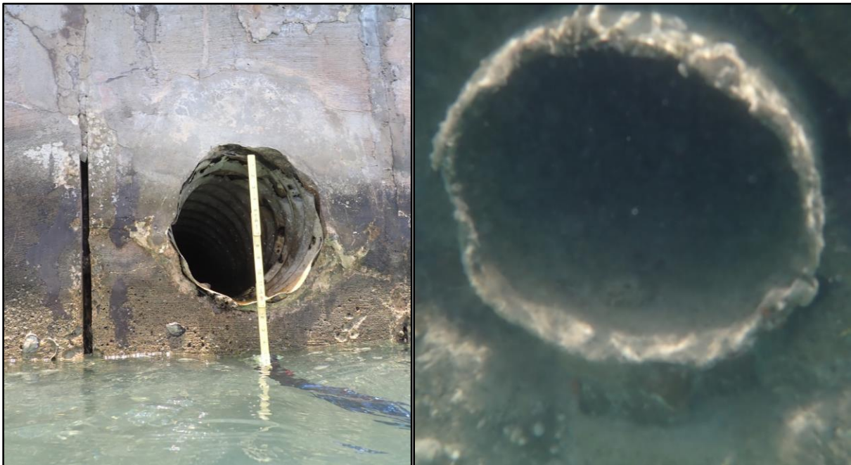
Photo 12: Typical corrugated metal outfalls at Section 4: 14 in. at STA 1+52 (left) and 10 in. at STA 4+09 (right)
