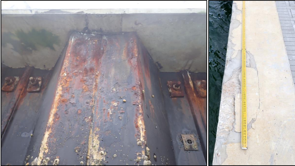
Photo 82: Typical condition of steel sheet pile and concrete cap STA 0+85 – STA 4+64
