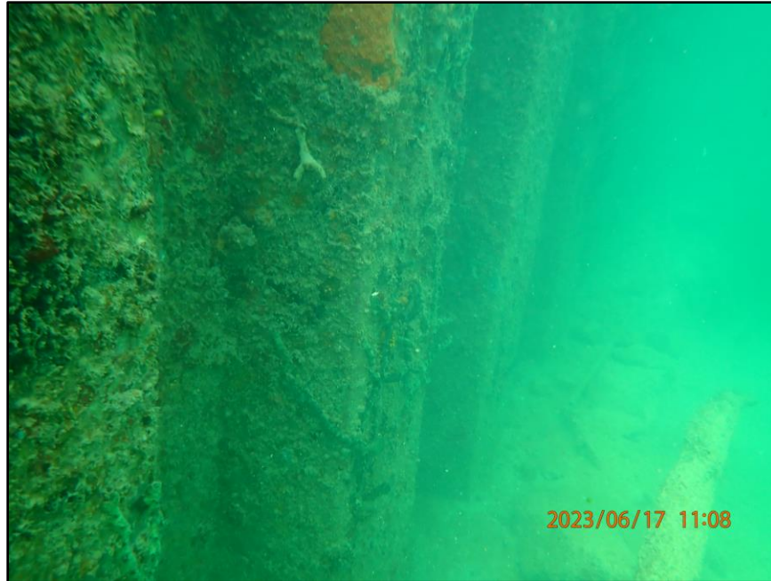
Photo 33: Original steel sheet piling along Section 11 northern bulkhead, STA 5+80 – 9+60
