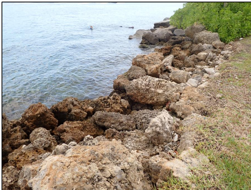
Photo 104: Localized areas of minor erosion of the upland fill
