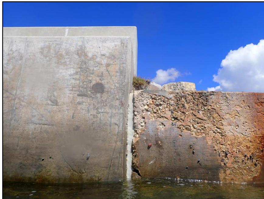
Photo 39: STA 0+00 Parcel 15 termination at Section 12
