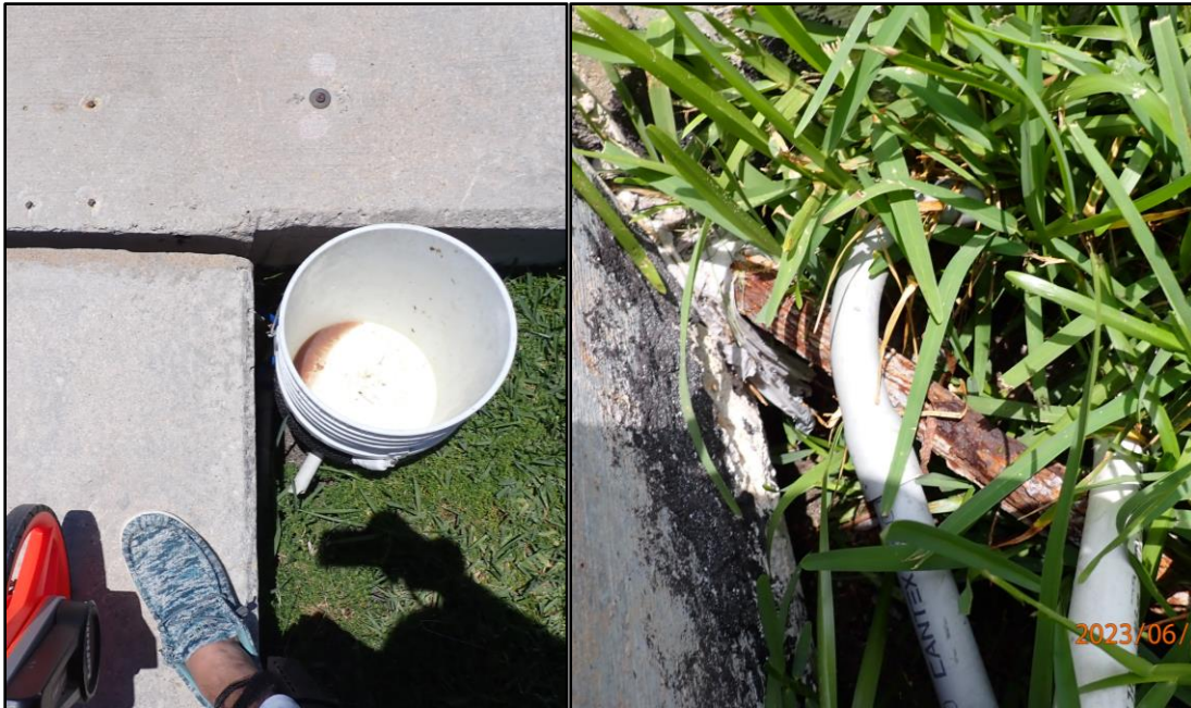
Photo 62: 1 ft deep sinkhole at Section 5 STA. 0+00 E (left) with exposed tie rod attached to Section 4 bulkhead (right)
