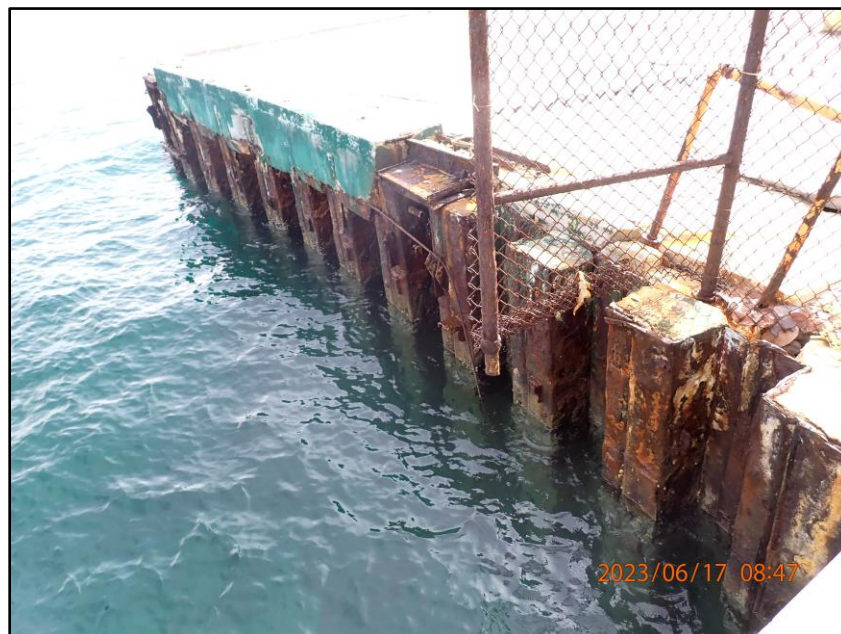
Photo 30: Typical view of northeast of Section 10 ferry basin bulkhead
