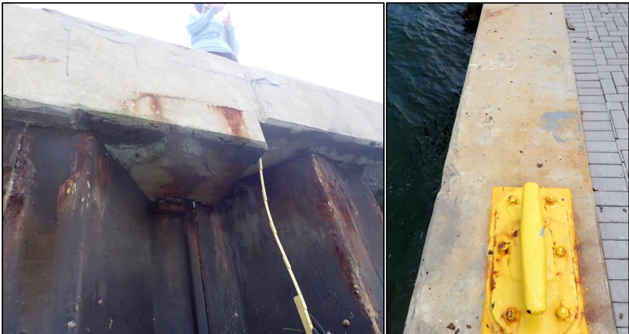
Photo 81: Typical condition of steel sheet pile and concrete cap STA 0+30 – STA 0+85
