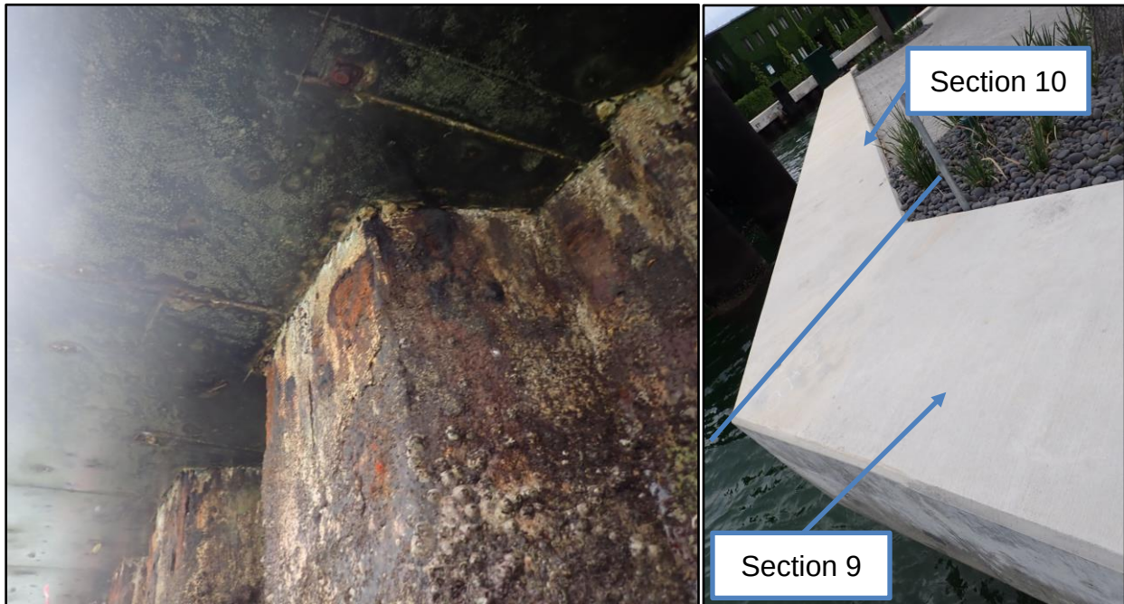
Photo 78: Typical condition of steel sheet pile (left) and concrete cap (right) STA 0+00 – STA 0+30
