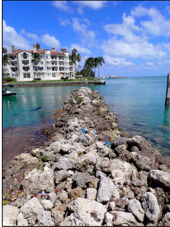
Photo 14: STA 2+80 view of Section 4 Southwest jetty at outlet of harbor
