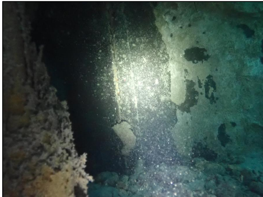
Photo 94: Typical steel surface of combi-wall with clean and intact coating
