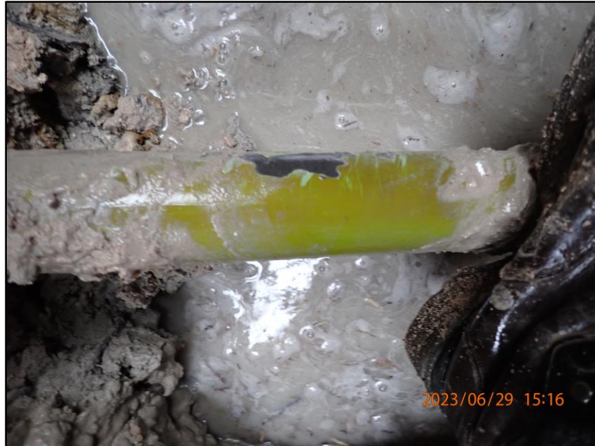
Photo 74: Tie rod inspected at STA 0+70 in like new condition
