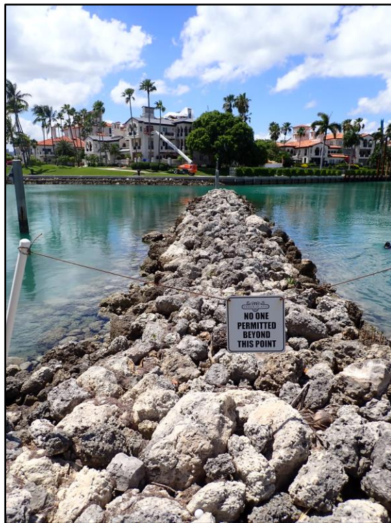
Photo 15: STA 2+60 view of Section 4 Northeast jetty at marina basin
