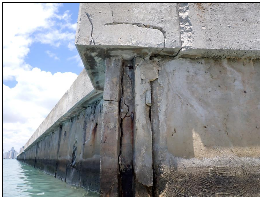
Photo 10: Eastern termination of Section 4 concrete sheet pile showing tongue-and-groove construction
