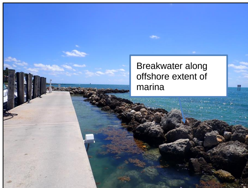
Photo 4: Section 2 breakwater along offshore side of Guest Marina, looking east
