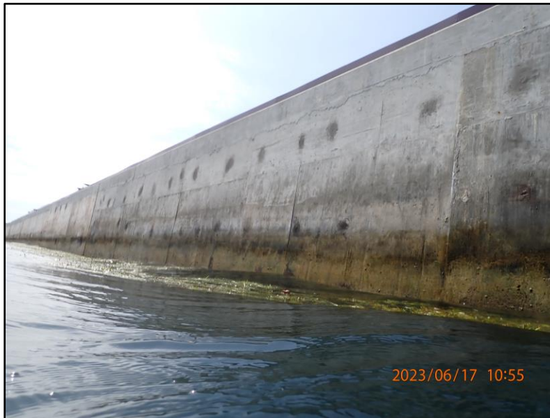
Photo 34: Typical construction of concrete cap throughout Section 11
