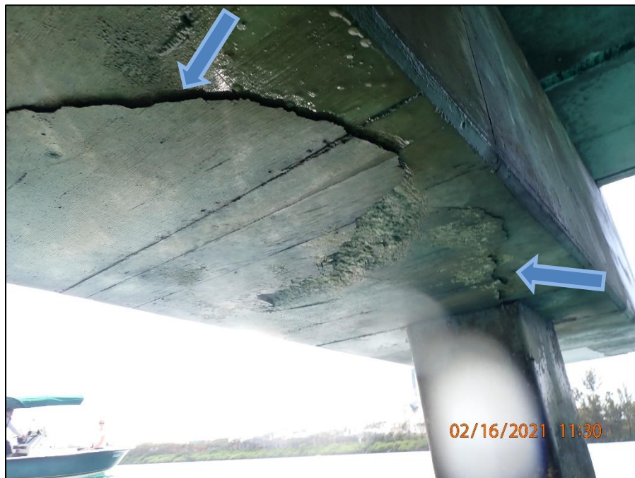
A.6: Concrete delamination along pile cap soffit between piles 7 and 8 at pile bent 1.
