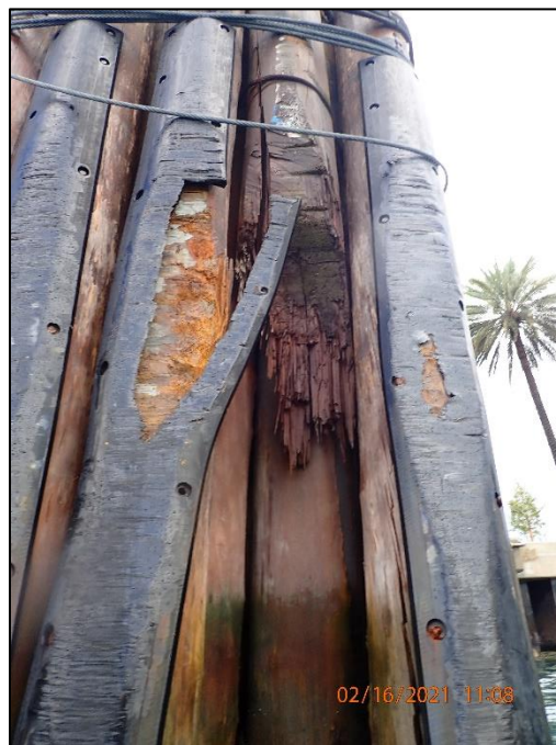
A.36: Southern face of west timber dolphin piling. Rubber fender pile damage and spilt pile observed within the ferry impact zone.
