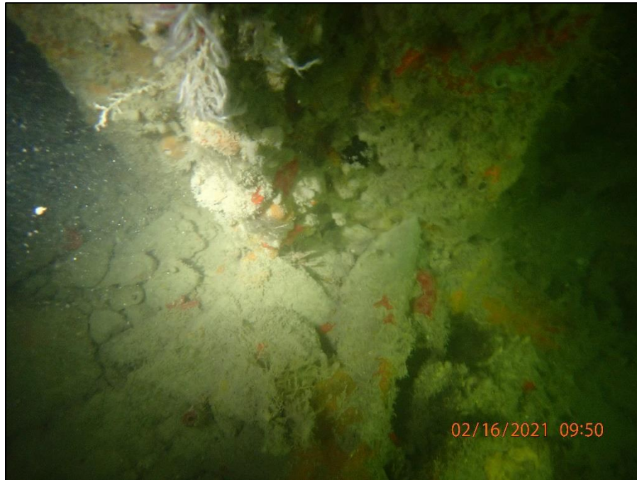
A.5: View of sheet pile bulkhead at the mudline. Note remnants of construction material and debris along the toe of the bulkhead.
