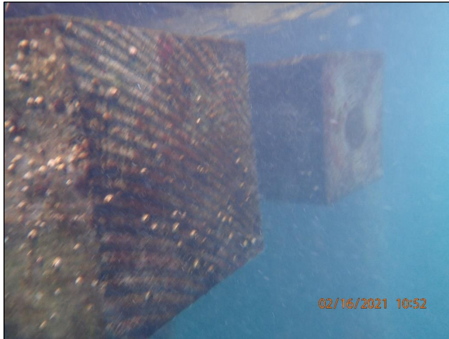
A.25: View bottom row of berthing dolphin timbers within tidal zone. Note no timber rot and minor marine growth.
