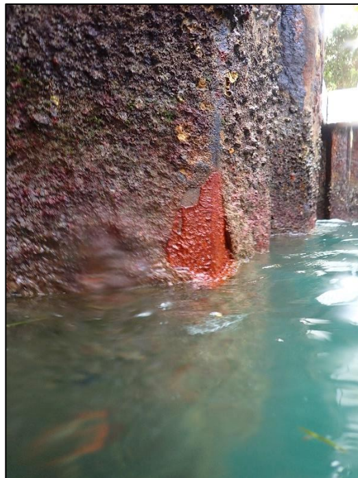
A.52: View of eastern bulkhead past southern hoist dolphin. Note soft erosion and section loss. Typical condition observed at the 4 th and 5 th sheet pile pairs south of the southern hoist dolphin and the 4 th -6 th sheet pile pairs west of the southeast corner of the bulkhead.
