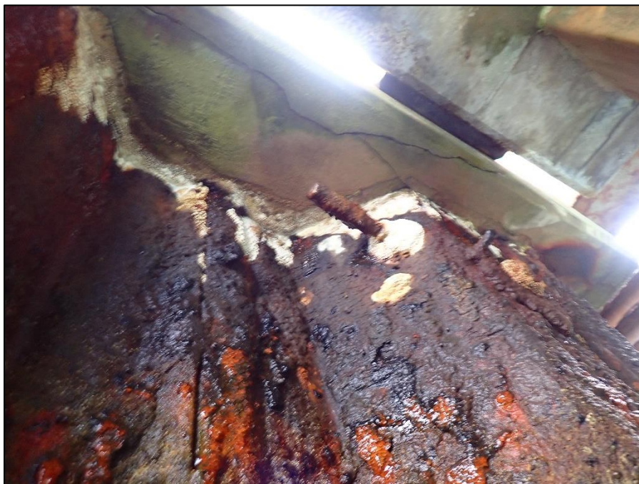
A.44: Eastern bulkhead at hoist dolphin connection to the concrete cap. Note cracking along the concrete soffit.
