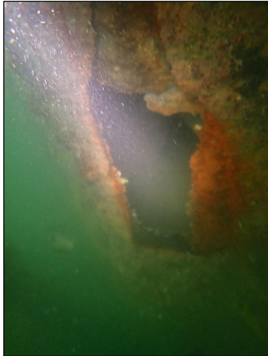
A.45: View of void through steel sheet pile wall approximately 2'x8" located halfway down the wall at the where the northern hoist dolphin meets the ferry ramp.
