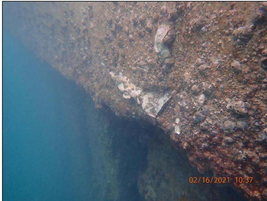
A.21: View berthing dolphins within the tidal and submerged zones. Note minor cap soffit spall and corrosion staining of concrete.
