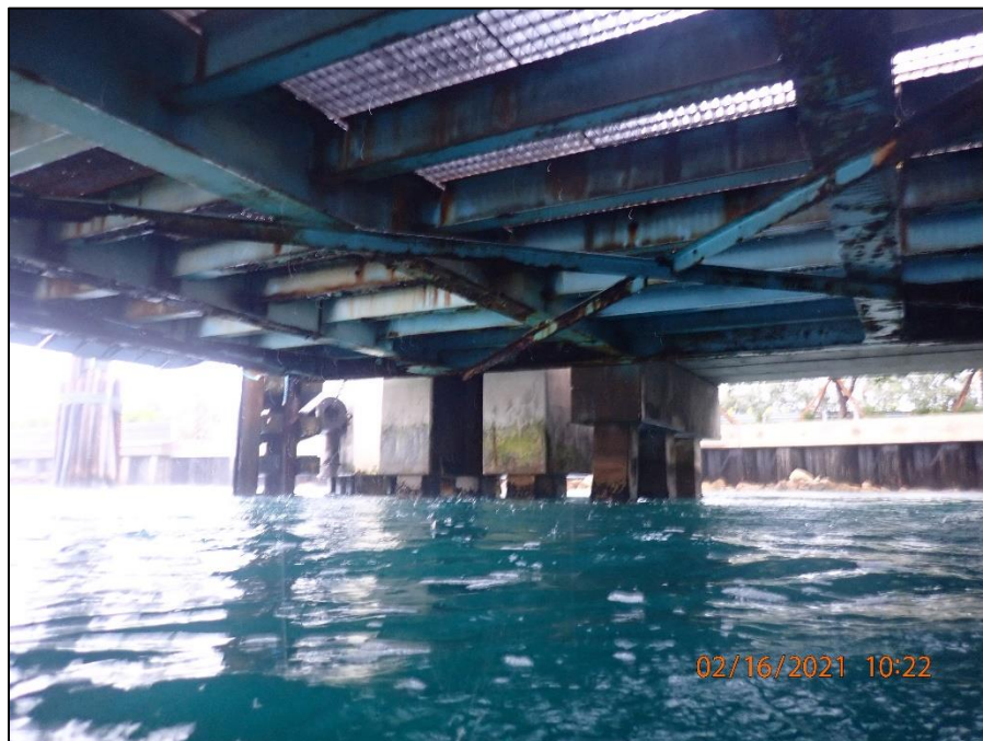
A.14: View of steel framing at wharf bridge with severe corrosion at the cross-bracing.
