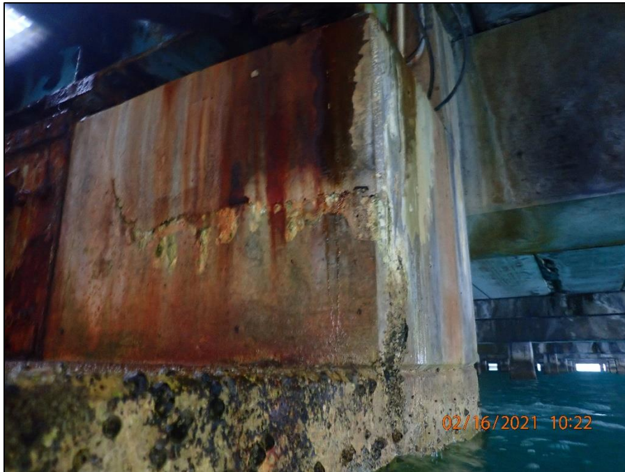
A.15: Concrete chemical deterioration, spalling, and corrosion staining at the bridge seat. Note steel beams from ramp secure to top of bridge seat.
