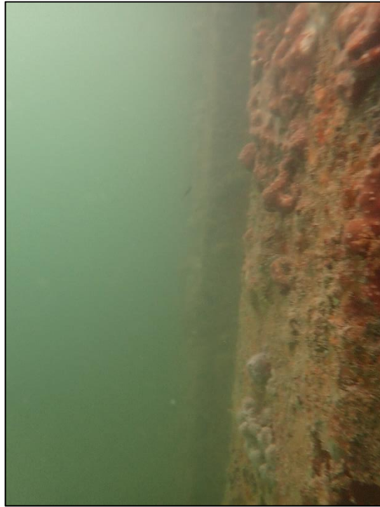
A.43: View of western bulkhead within tidal and submerged zone. Note corrosion of sheet piles and marine growth.
