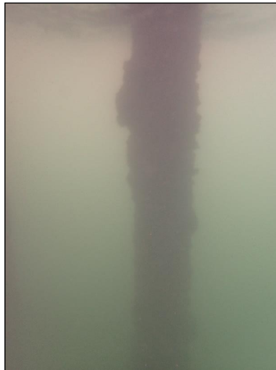
A.62: View of berthing dolphin steel pipe pile within the tidal and submerged zone. Note corrosion and marine growth on pile.
