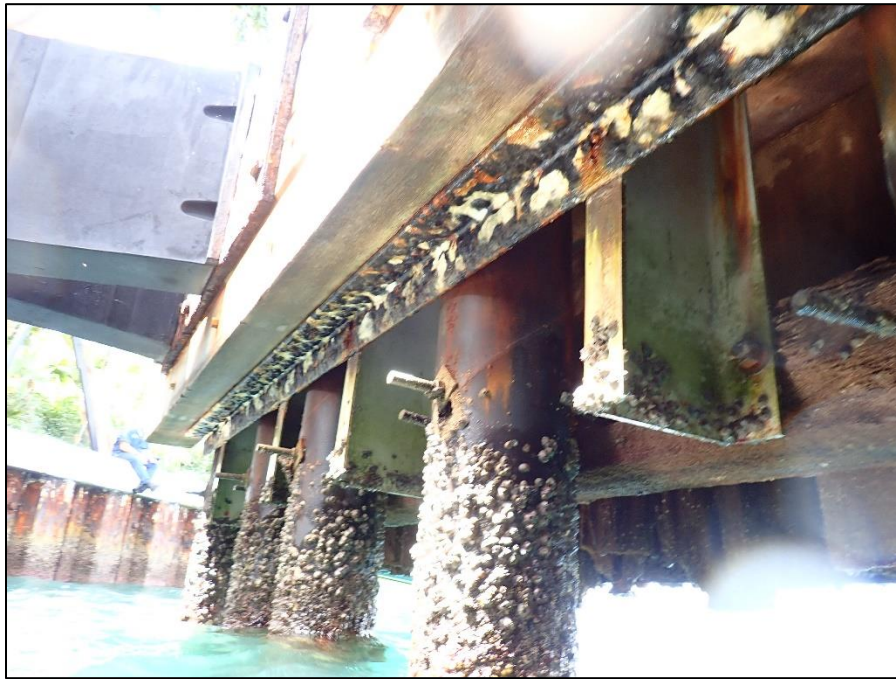
A.61: View of corrosion and marine growth within the splash zone for steel pipe piles and aluminum channels at the berthing dolphins.
