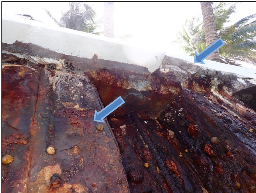
A.56: View of spalling along the concrete cap soffit along the eastern bulkhead at the 2 nd sheet pile pair from the ladder. Note sheet pile corrosion scaling, typical within inspection scope.
