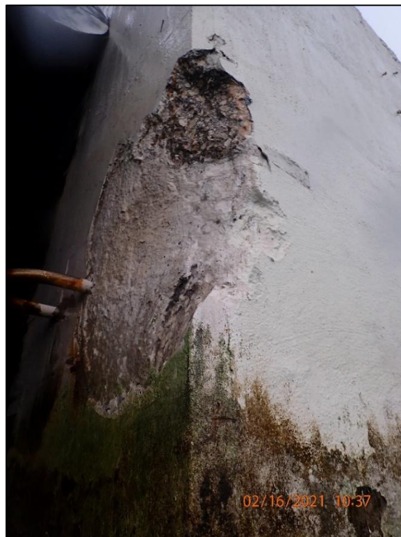
A.20: View of concrete spall on southern face of south berthing dolphin.
