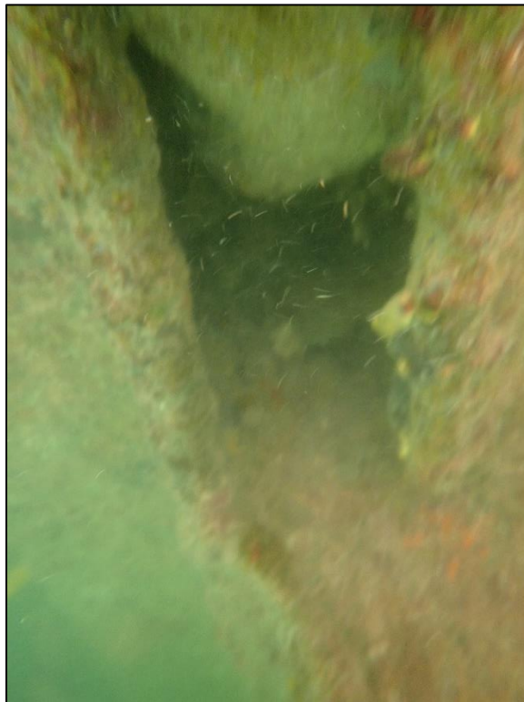
A.48: Cavity through steel sheet pile located at northern hoist dolphin and ferry ramp connection.
