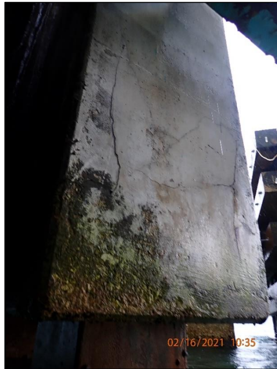
A.17: Concrete delamination on northern face of north hoist dolphin.
