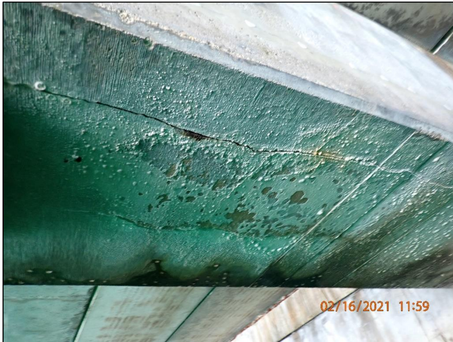
A.11: Typical cracking along pile cap soffit with minor concrete delamination.
