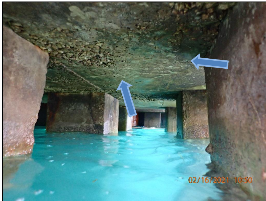
A.31: Typical concrete cracking at the berthing dolphin cap soffit.
