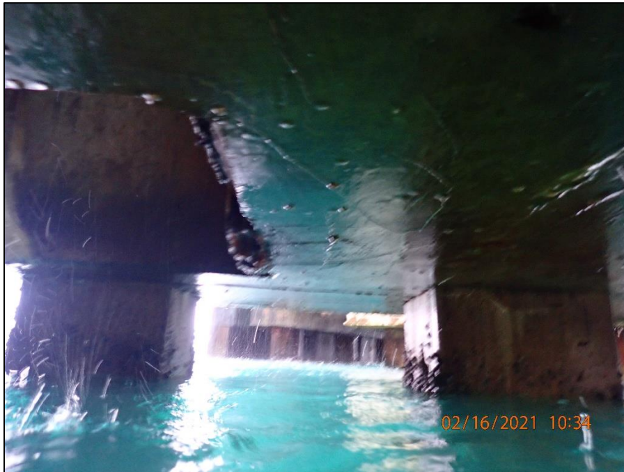
A.19: View of concrete cap soffit at hoist dolphin with typical concrete cracking.
