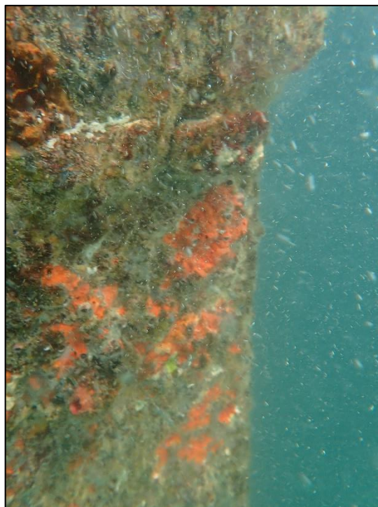
A.66: View of jacketed section of hoist dolphin pile end within the submerged zone. Note pile observed to be satisfactory below the pile jackets.
