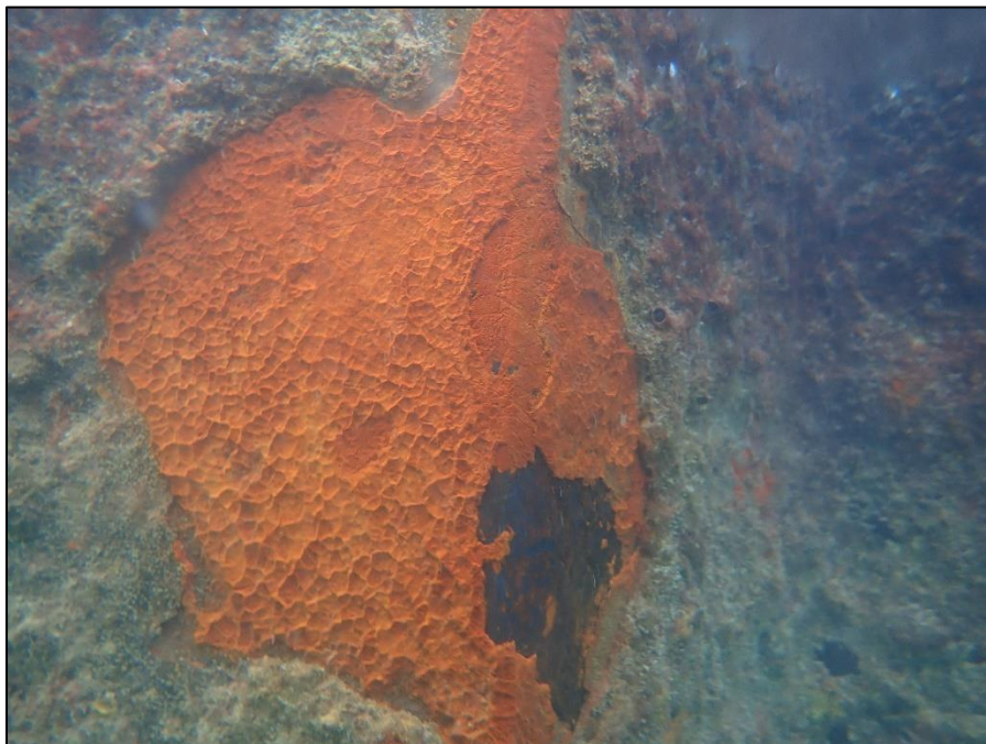
A.54: View of soft chemical deterioration and section loss of sheet pile within the tidal and low water zones.
