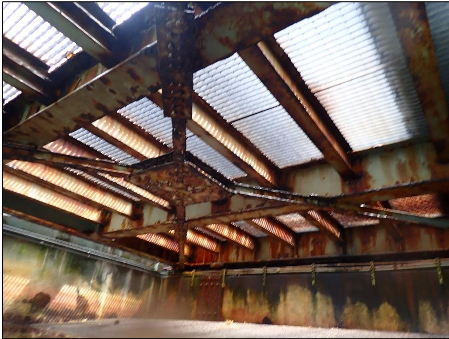
A.49: View of ferry ramp support. Note corrosion of steel beams and cross-bracing. Cross-bracing severely corroded.
