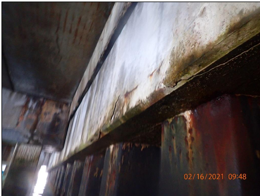
A.2: Typical concrete cracking along the wet face and soffit of the bulkhead cap.
