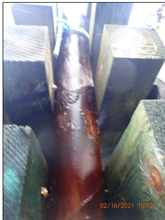
A.24: View of berthing dolphin timber fender system. Note corroded steel pipe piles.
