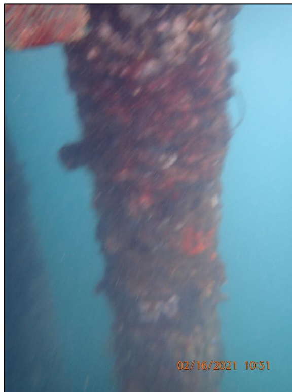
A.26: View steel pipe piles of berthing dolphins within tidal and submerged zone. Note steel corrosion and marine growth.
