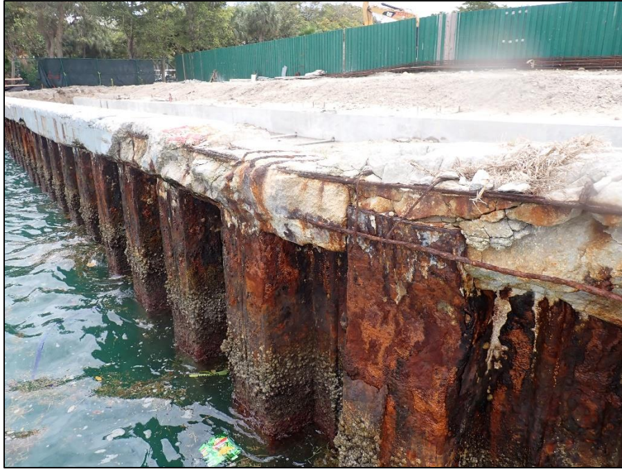
A.37: View of western-most corner of bulkhead within inspection scope. Note deep cap spalls exposing reinforcing steel and corroded steel sheet pile.
