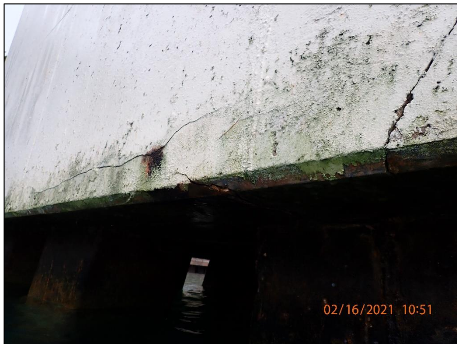
A.32: Typical concrete cracking of berthing dolphin pile cap edges.
