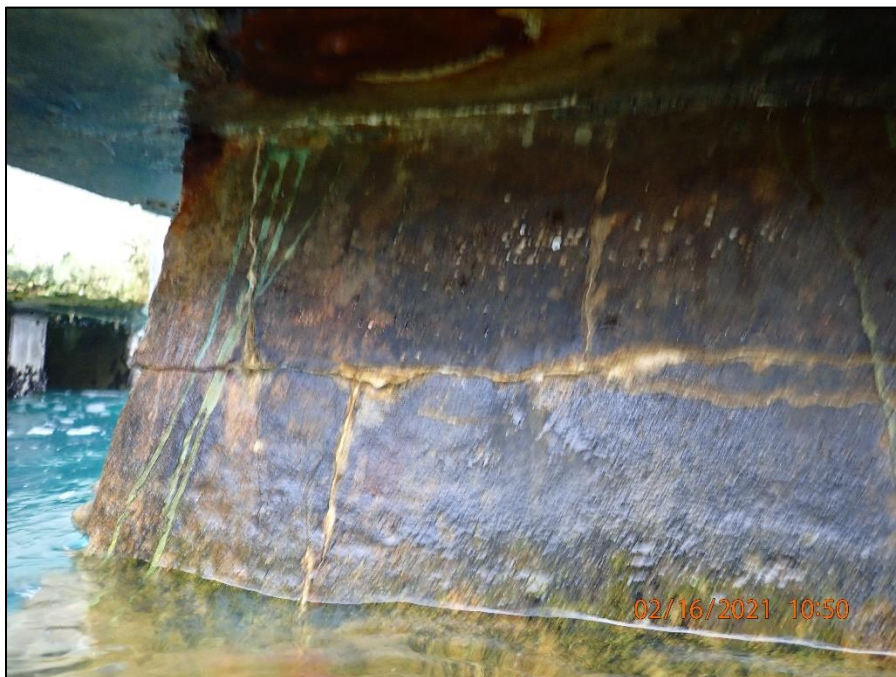
A.30: Typical concrete cracking of berthing dolphins piling.
