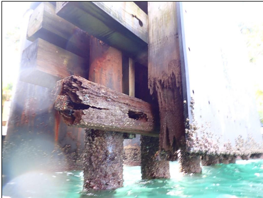
A.60: View of timber rot at bottom timber and timber fascia on the berthing dolphin. Typical condition for both north and south berthing dolphins.
