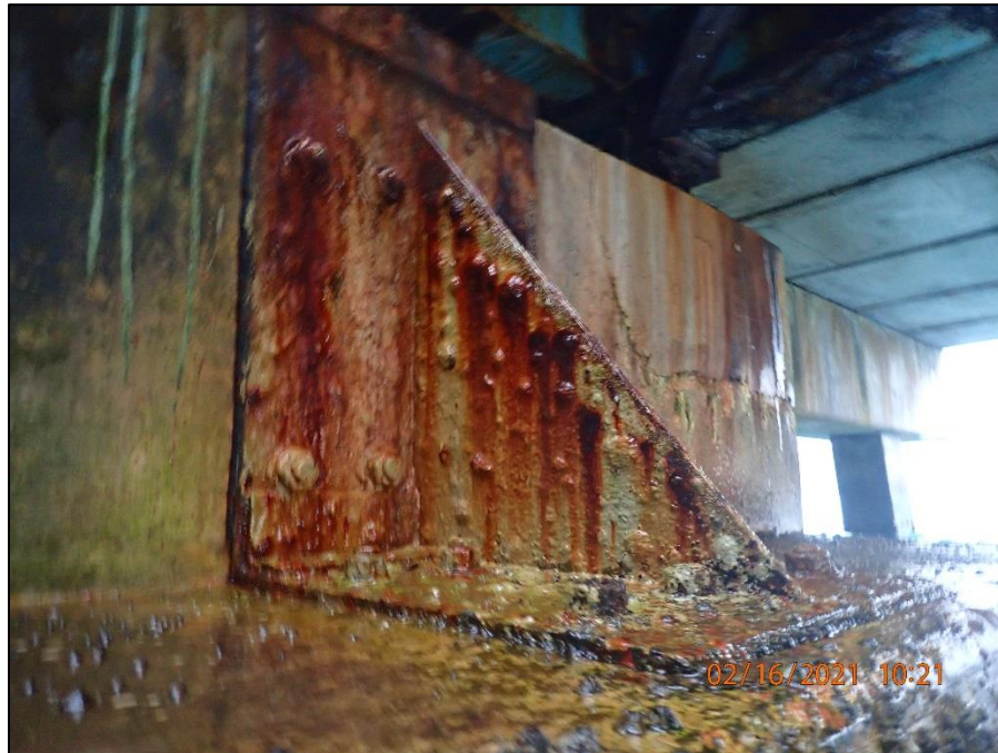
A.13: View of corrosion at the steel gussets at the wharf bridge seat.
