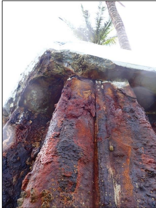
A.57: View of spalling at concrete cap at southern corner of bulkhead. Note exposed reinforcement in concrete cap and steel corrosion staining in cap.
