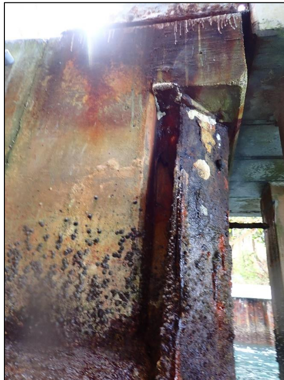
A.50: View of eastern sheet pile connection to southern hoist dolphin. Note connection appears generally intact.
