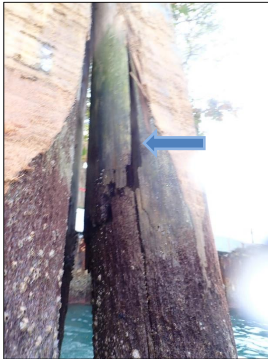
A.67: View of typically observed flexural failure of the timber piles in the timber dolphin. Note northern face damage of piles within the impact zone of the dolphin.
