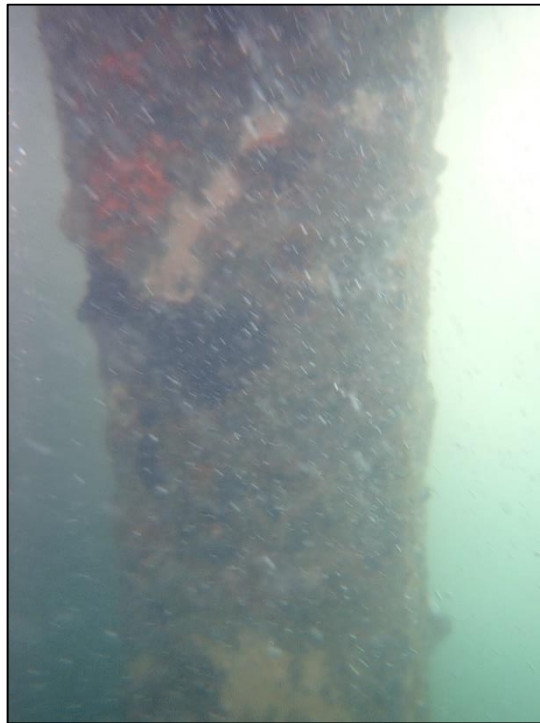
A.65: View of jacketed hoist dolphin piles within the tidal and submerged zone. Note pile observed in good condition with pile jackets.
