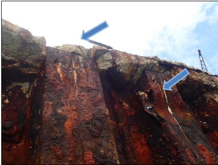
A.39: View of western bulkhead at 20 th sheet pair or approximately 75 feet east of the most west bulkhead corner. Note damage in sheet pile causing void in sheet. Note cap spalled off.
