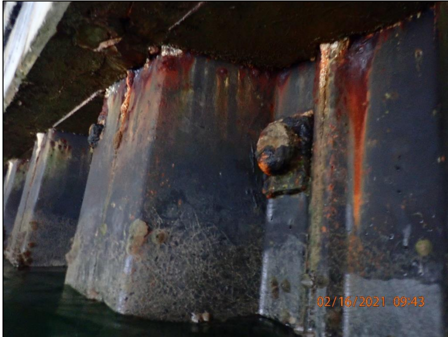
A.1: View of steel sheet pile exhibiting minor corrosion at the steel sheet pile and anchor heads.
