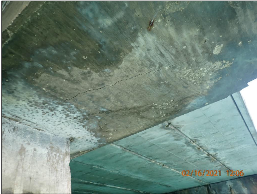
A.9: Typical cracking at cap soffit observed adjacent to concrete pile head connection to cap.
