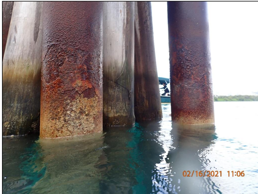
A.33: Corrosion at the steel pipe piles in splash zone at eastern timber dolphins.
