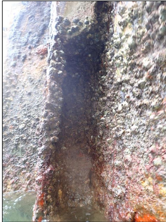
A.53: View of sheet pile wall void within the splash zone.
