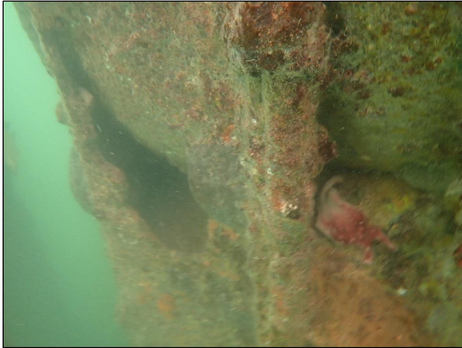
A.47: View of cavity through steel sheet pile located where the northern hoist dolphin and ferry ramp meet.
