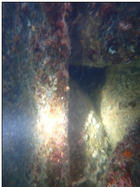
A.46: View of cavity through steel sheet pile at the connection between the sheet pile wall at northern start of the ferry ramp wall.
