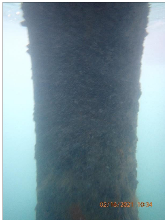
A.18: Typical hoist dolphin concrete pile in the tidal zone. Note minimal section loss of piles.
