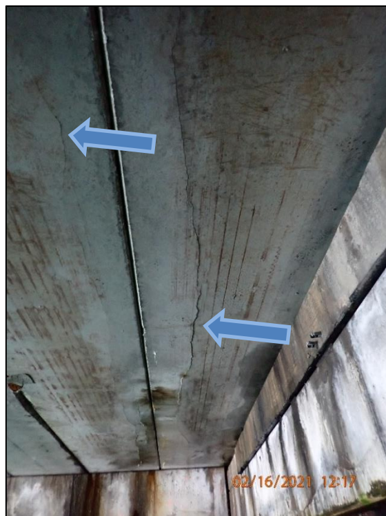
A.28: View of cracking along concrete deck soffit.
