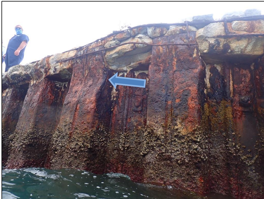
A.38: View of western-most corner of bulkhead within inspection scope. Note damage to steel sheet just below concrete cap, corrosion and marine growth in the splash zone.
