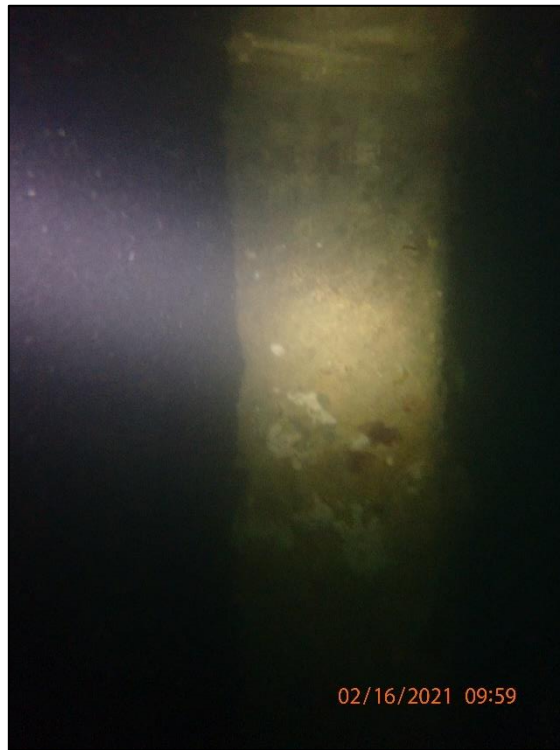
A.8: Typical concrete pile within tidal and submerged zone. Note minimal section loss.
