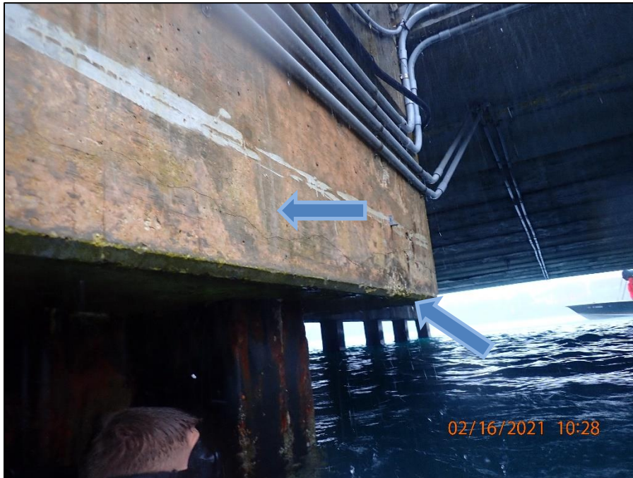
A.3: View of concrete spall and cracks in bulkhead cap adjacent to pile bent 4.
