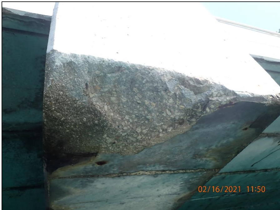
A.10: Spalling at concrete pile cap observed on the south face of pile bent one.
