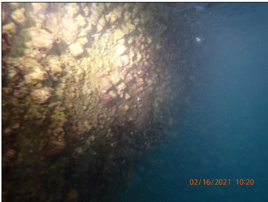
A.16: View of bridge seat pile cap within tidal zone. Note marine growth on concrete and minor corrosion staining.
