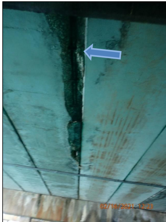
A.27: View of spalling at the concrete deck soffit.
