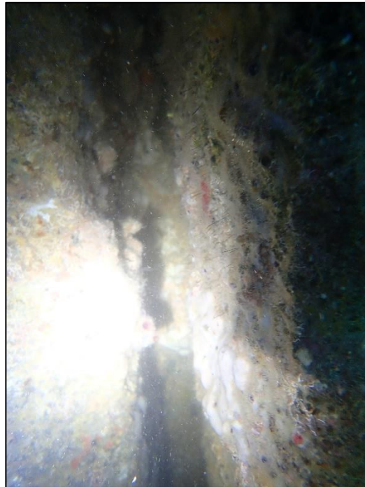
A.51: Underwater view of sheet pile wall connection with ramp wall at the southern hoist dolphin. Note seal appears to be generally intact and cavities were not observed at the time of inspection in this location, unlike the northern hoist dolphin sheet pile and ramp wall connection.
