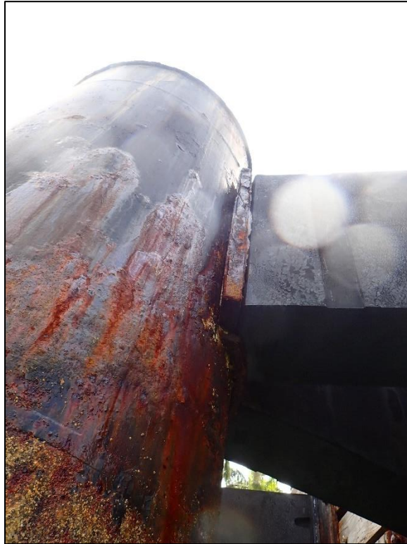
A.59: View of steel pipe pile approximately 48” in diameter at the berthing dolphins. Two piles were observed for each berthing dolphin. Note corrosion in the splash zone.
