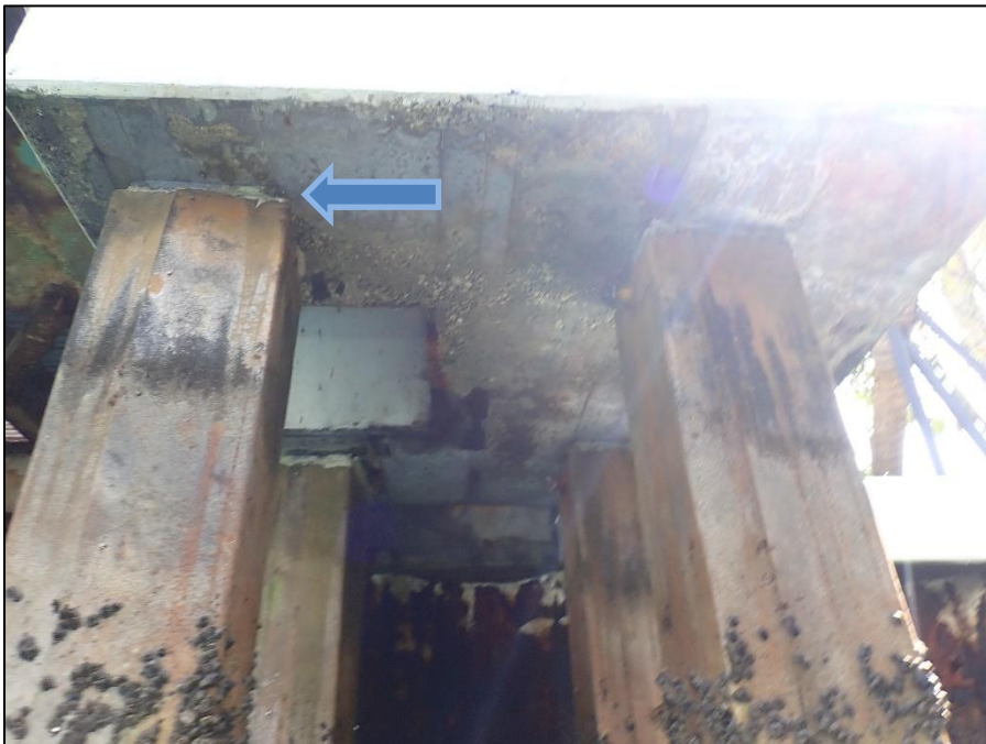
A.64: View of hoist dolphin. Note pile jackets on concrete piles.
