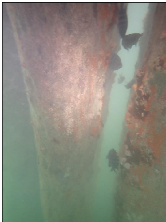
A.68: View of timber dolphin piles within the submerged zone. Minimal section loss of timber piles was observed.
