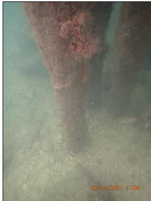
A.35: View of timber dolphin piling at mudline. Note typical section loss of about 50% near mudline.
