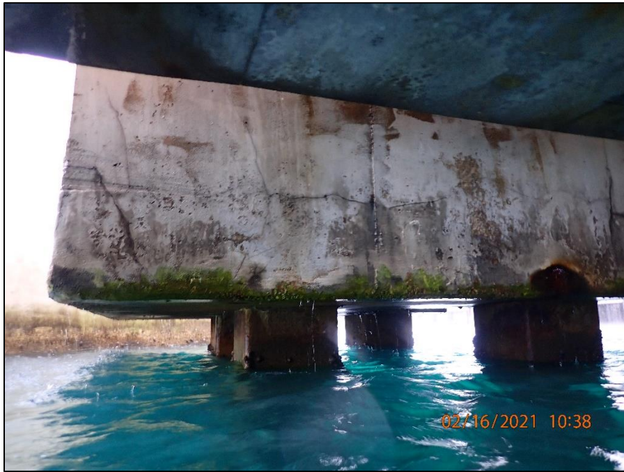
A.29: View of pile cap cracking at spanning across multiple piles in the bent.
